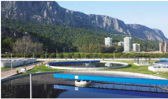
REMONDIS develops and operates facilities to treat wastewater and produces high quality process water for its industrial customers
