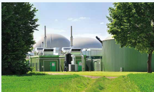
We help our industrial customers to generate biogas from their wastewater – from planning the concept all the way through to delivering it
